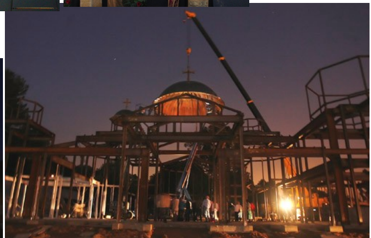
Like a flying saucer in the night, the main dome was raised and set in place - a spectacular sight that the many parishioners of St. Andrew church who witnessed the event will not soon forget.
